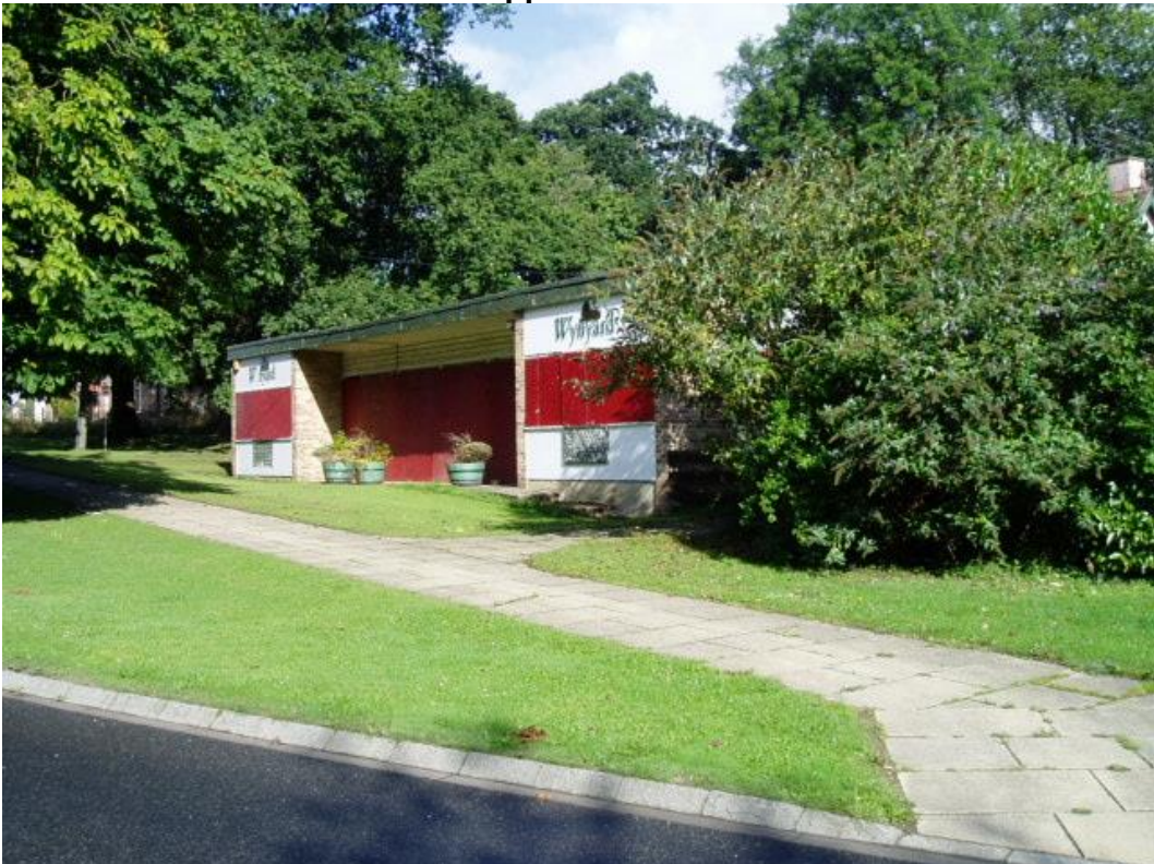
Appendix. 6b – View of former estate offices
